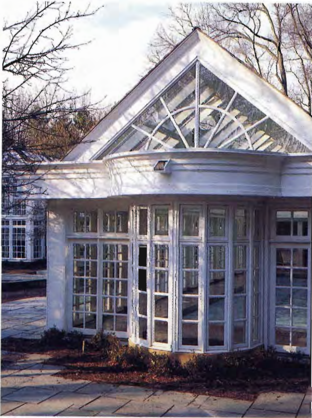
A CLASSIC SEMICIRCLE OF WINDOWS CURVES AROUND THE SPA AT THE TERMINUS OF THE NEW POOLHOUSE; THE CASEMENTS OPEN FOR VENTILATION.
